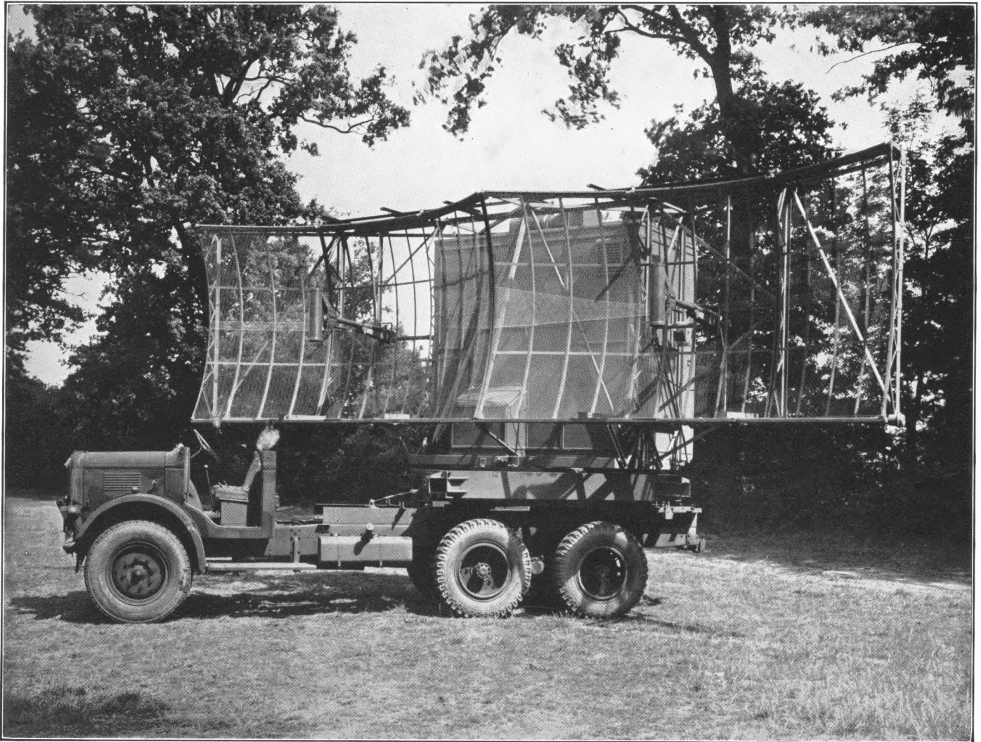
AMES Type II Mk. II (M). Prime-mover Aerial/Transmitter Vehicle (RV 433) only
